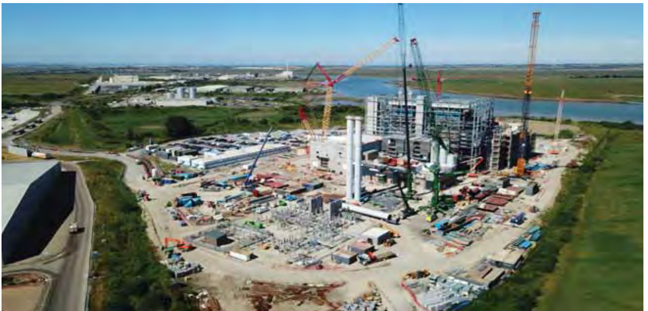
Figure 3: K3 facility under construction in July 2018
