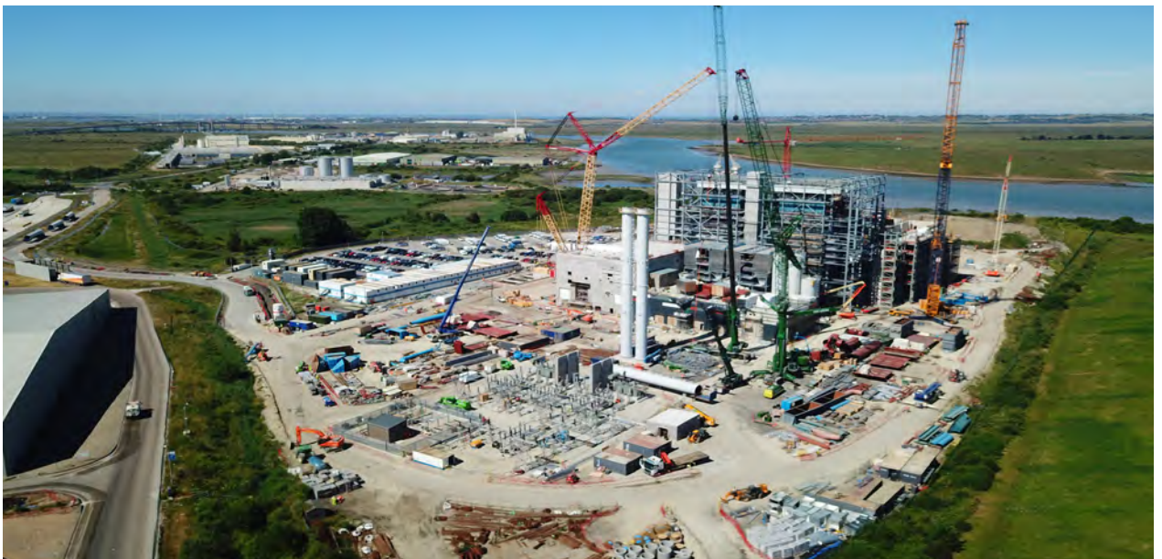
Figure 3: K3 facility under construction in July 2018
