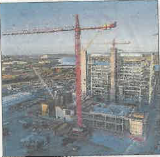
Construction started in 2018 but the firm hopes to expand
