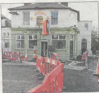
The pub is already facing disruption from roadworks
